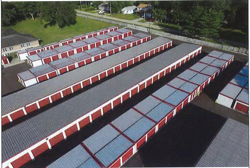
This project features micro systems with Iced White walls and Garnet doors. Units are placed on asphalt to expand rentable square footage of existing facility.
