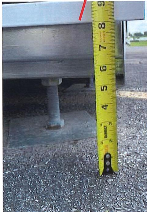
On the low side you will unscrew the leveling feet to make sure the unit is level. There is 6" of play in the leveling feet.
