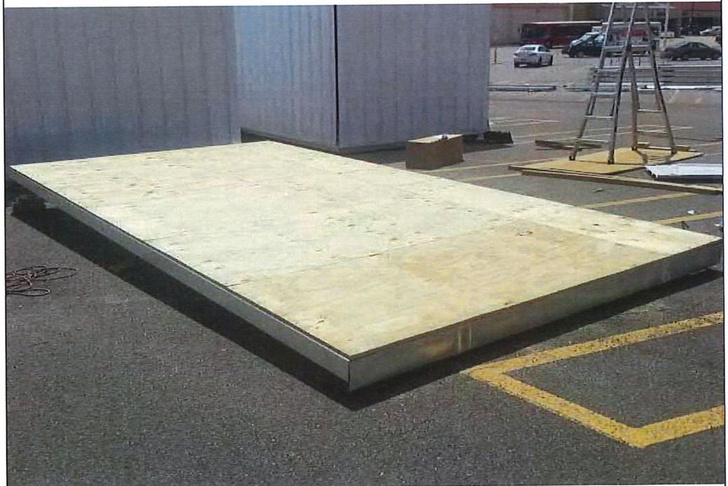
The floor system is leveled by using leveling feet when installing the structure.
